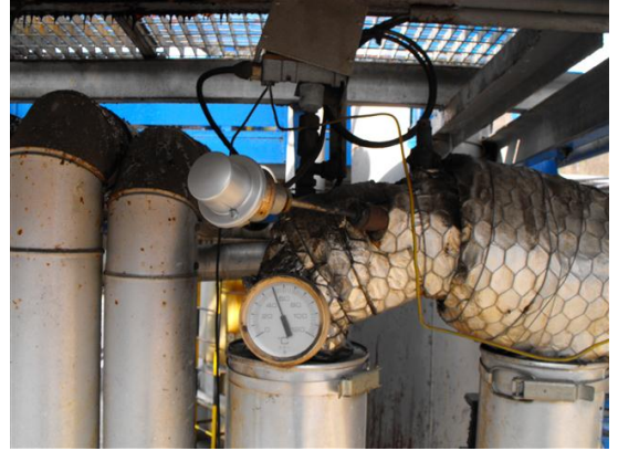
(b) Temperature sensor of supply water.
